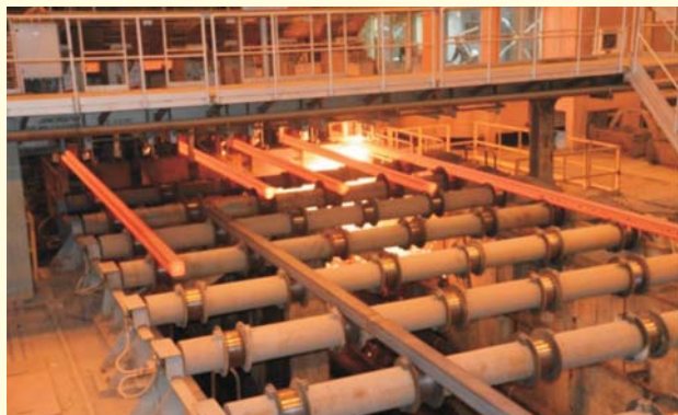
Highly energy efficient Continuous Caster at ISP
