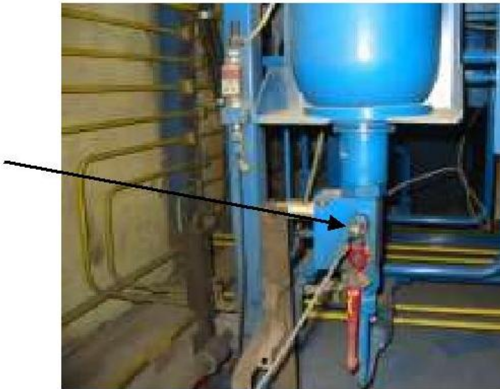
ARROW IN THE PICTURE IS SHOWING MINIMESH POINT FIGURE- 4
