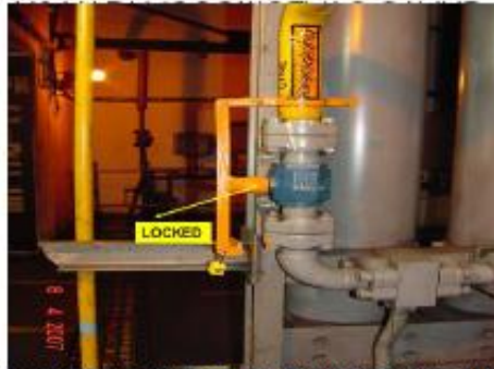
Arrangement made to lock hydraulic line ball valve at HSM
