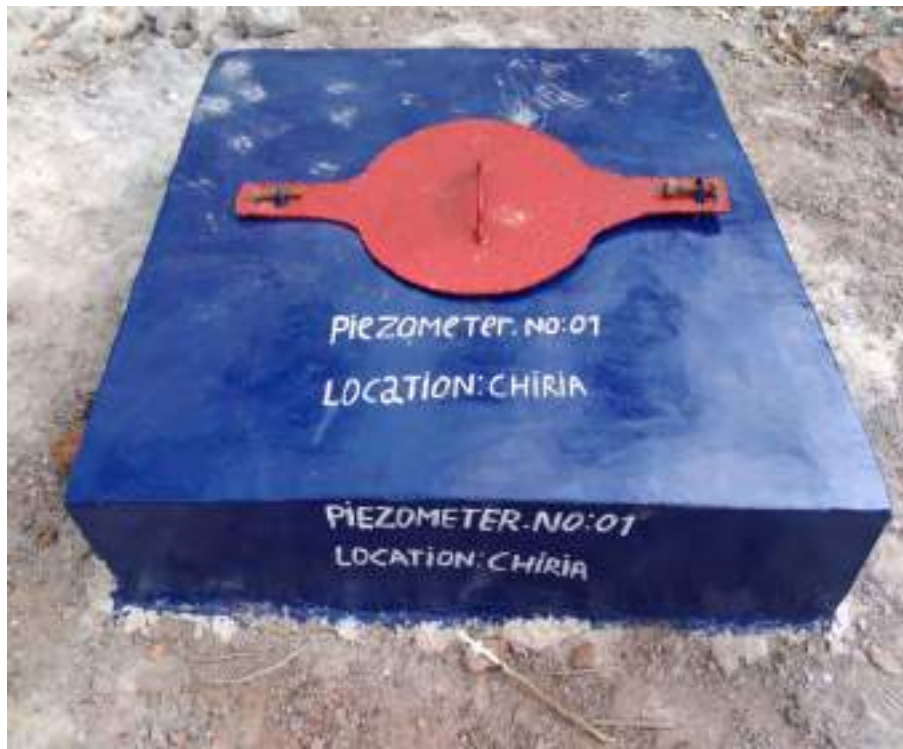
1. Piezometer at Chiria Village
