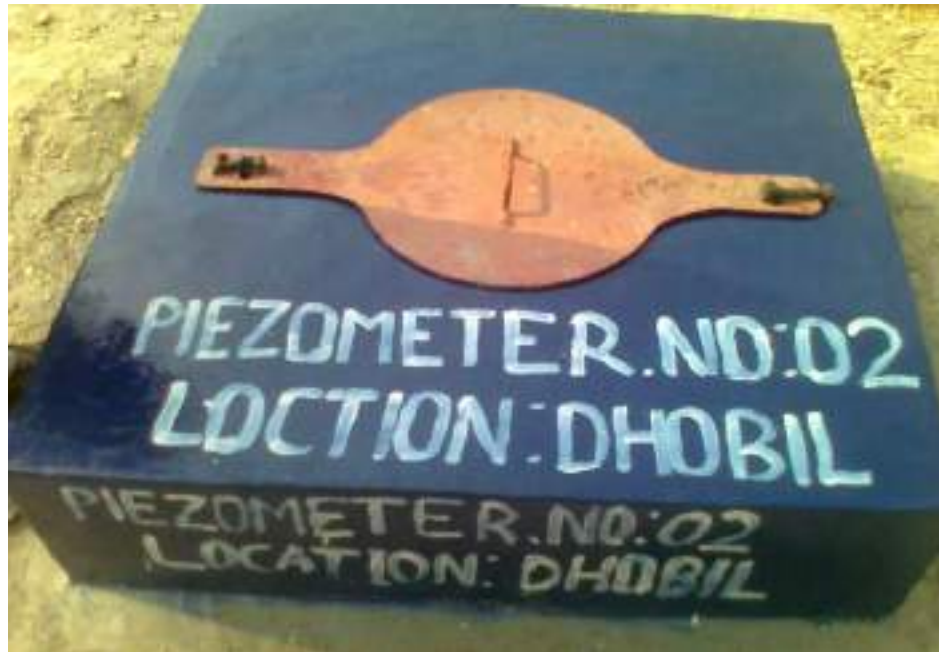
2. Piezometer at Dhobil Village
