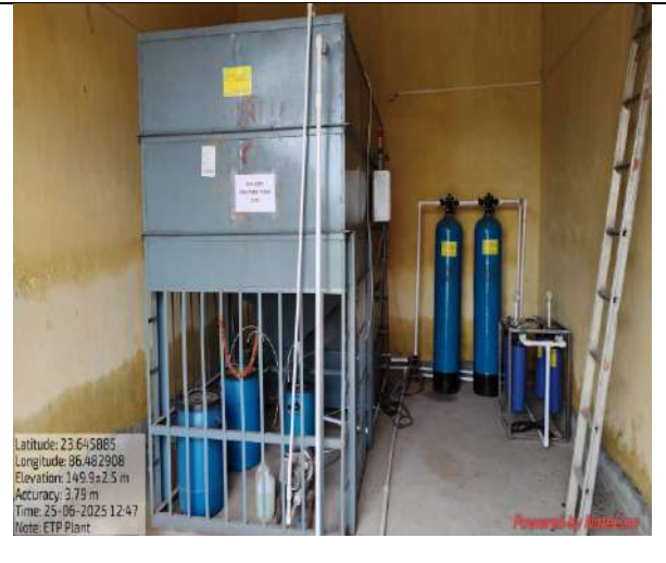
ETP installed at Project site
